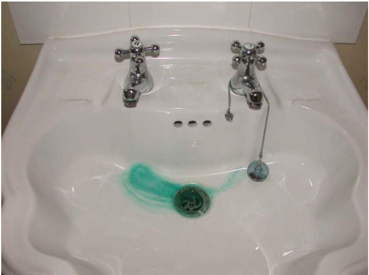
*Figure 5b Staining in hand basin caused by blue water.*
