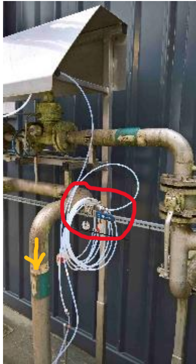
Figure 31: Product gas intake position before receiver station at Solrød Bioenergy (red, pressure around 5 bar). Flow direction is given by yellow arrow.
