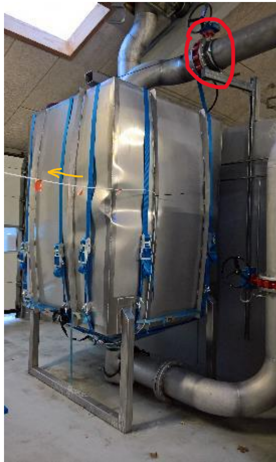
Figure 21: Biogas in-take location after VOC filter (red line). Arrow shows direction of the gas flow to the tent.
