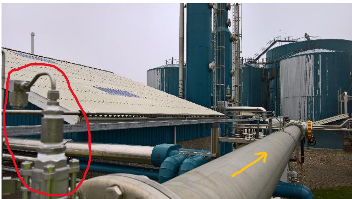
Figure 27: Raw-biogas in-take location before amine adsorber and gas flow direction (red circle and yellow arrow, respectively).
