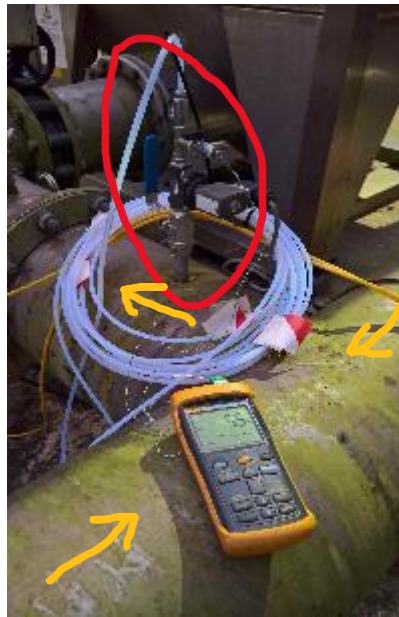
Figure 40: Raw biogas intake position (red, pressure a bit above 1 bar, temperature about +5.5°C). Flow directions are given by yellow arrows.
