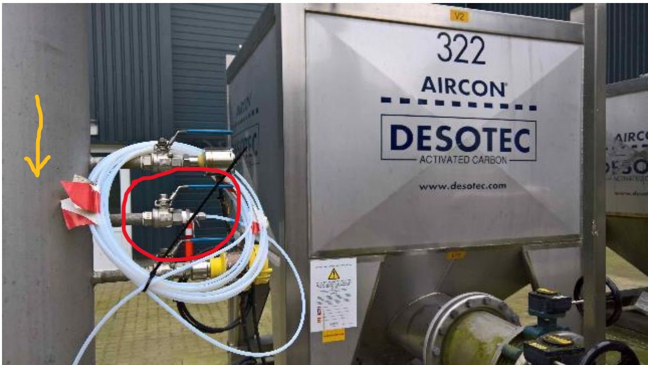
Figure 35: Biogas intake position after VOC filter (red, pressure a bit above 1 bar). Flow direction is given by yellow line.
