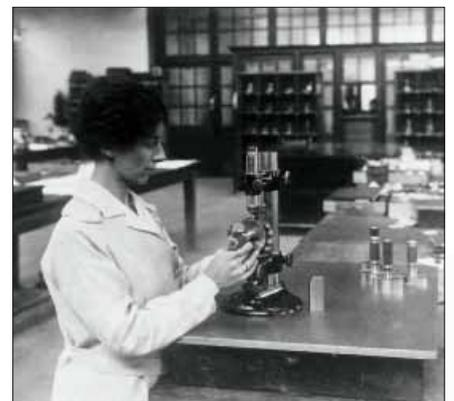
NPL testing gauges used in the manufacture of fuses and shells during the First World War.
