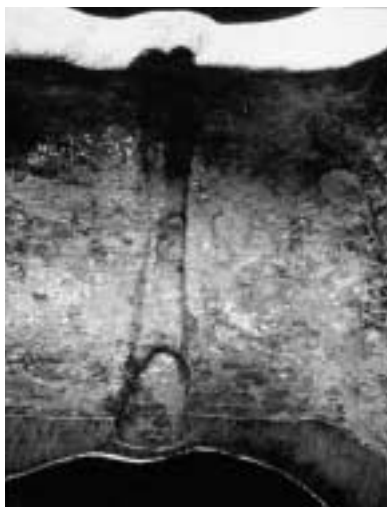
Figure 5. Preferential corrosion of a weld in a carbon steel pipe
